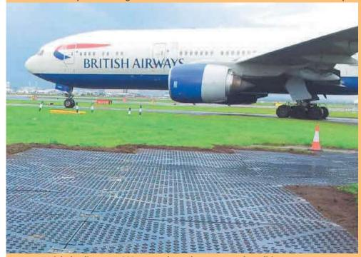
Weight loading up to 200 tonnes dependent on ground conditions
